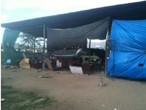
Existing Temporary Classroom Villa
